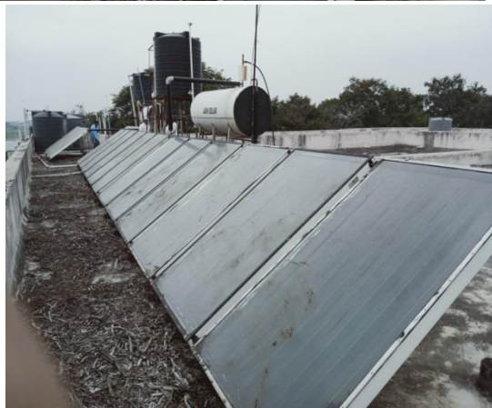
*Solar Energy Plant for Hot Water System in Ladies Hostel
